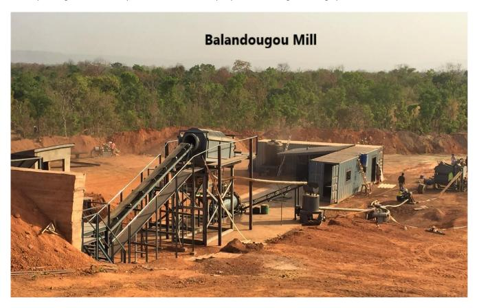
The 150 tpd gravity mill production line includes a 5 tonnes upper feeder bin feeding a 40 tph vibrating feeder, a primary crusher, a cylinder washing machine, secondary fine crusher, a ball mill and two S-60 Knelson concentrators with capacity to process each up to 35 tph of wet material at a 50- 60% density.
