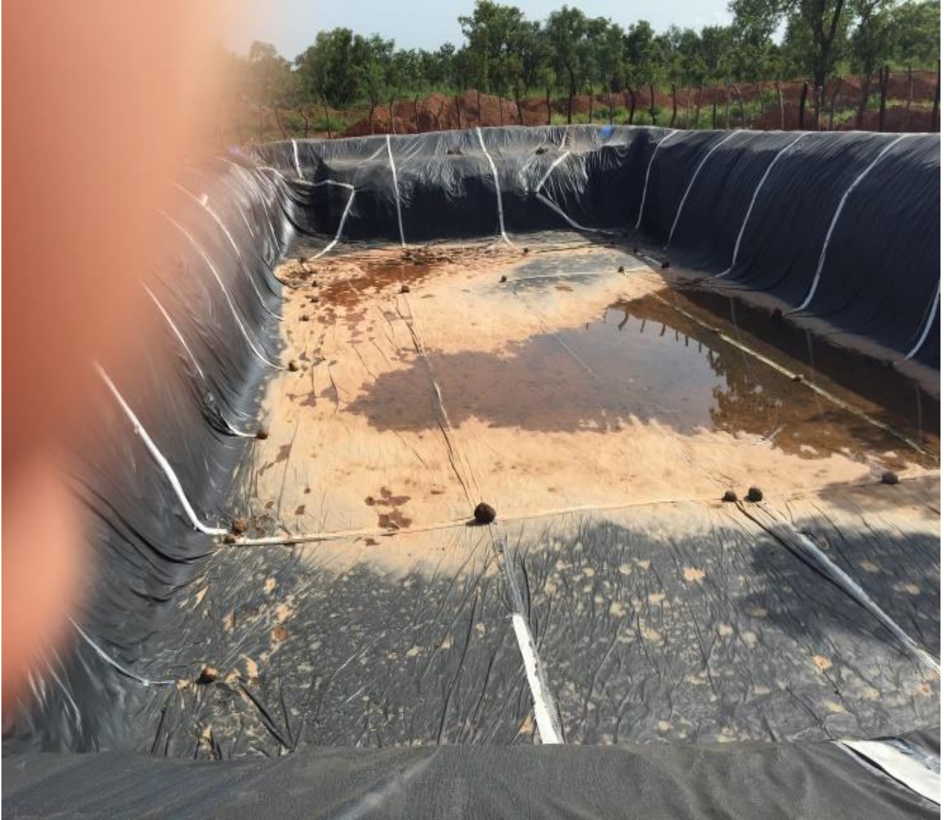
Picture 6 - 1.5 million litre water reservoir before filling
