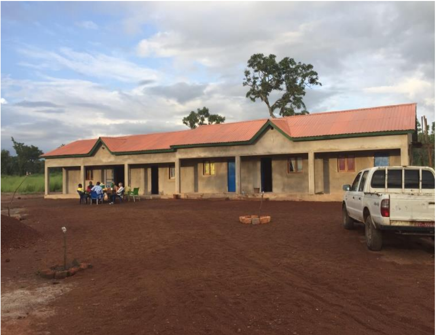
Picture 5 - Staff Camp Site - Building 1 (staff accommodation and office) of 5 buildings total. The mill camp has sleeping accommodation for up to 12 people.
